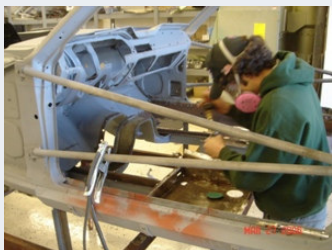
Justin cleaning up for new floor pan installation.
